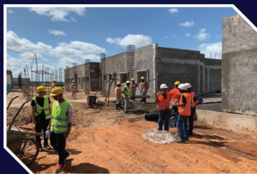
Construction works at Namacurra, Mozambique
